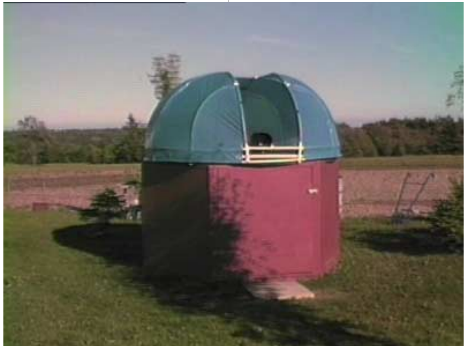
Current state of Observatory after painting and putting in a floor
