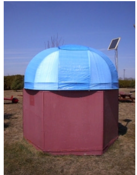
A view of the observatory with the solar panel installed
