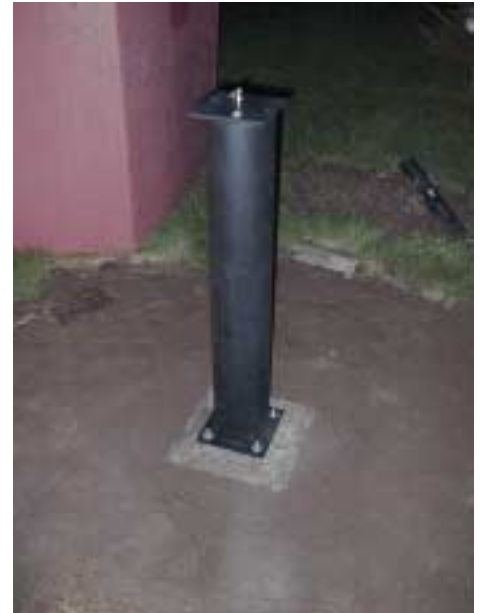
New pier mounted on the cement base.
